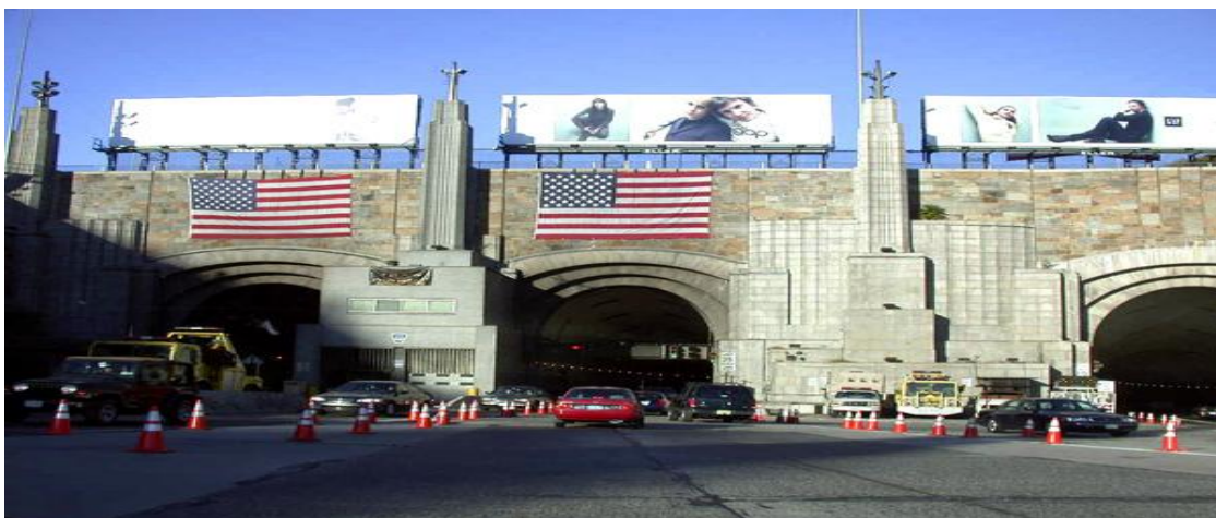
Figure 2: Lincoln Tunnel, New York Source: Lincoln Tunnel (2010)
