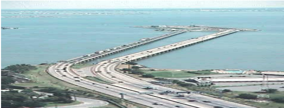
Figure 3: Hampton Road Bridge-Tunnel, Norfolk Source: Scott N. Kozel (2011)
