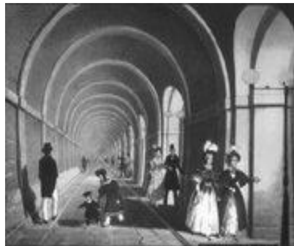
Figure 2: Thames Tunnel, London, 1843 Source: (Groves, G. L 1843)
