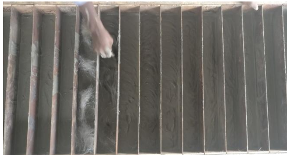
Fig2. Casting of foam concrete beams using glass fibre.
