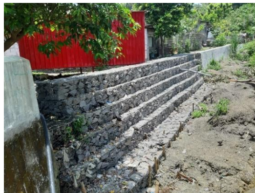
Figure 9: Wire gabions (October 2024)
