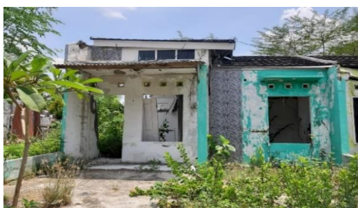
Figure 2. Affected houses (October 2024)
