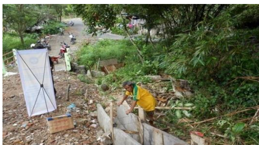
Figure 6: Road repair activities (October 2024)
