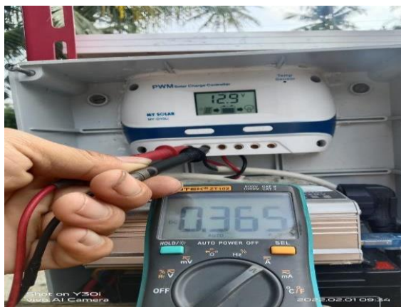
Figure 8. Current measurements using a multimeter
